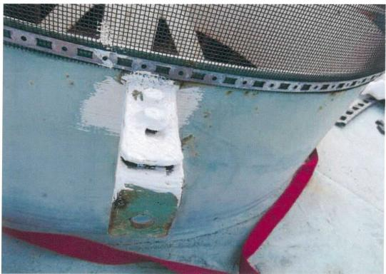
Roof vent cover bracket after spot repair. One of the three brackets had completely corroded and was no longer attached. The vent is held in place with the two remaining brackets.
