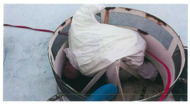
Corrosion removal in process on rafters inside of roof vent.
