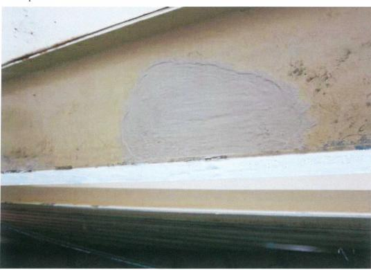
Typical spot repair on roof support rafter on tank interior. Approximately 100 similar locations were repaired.
